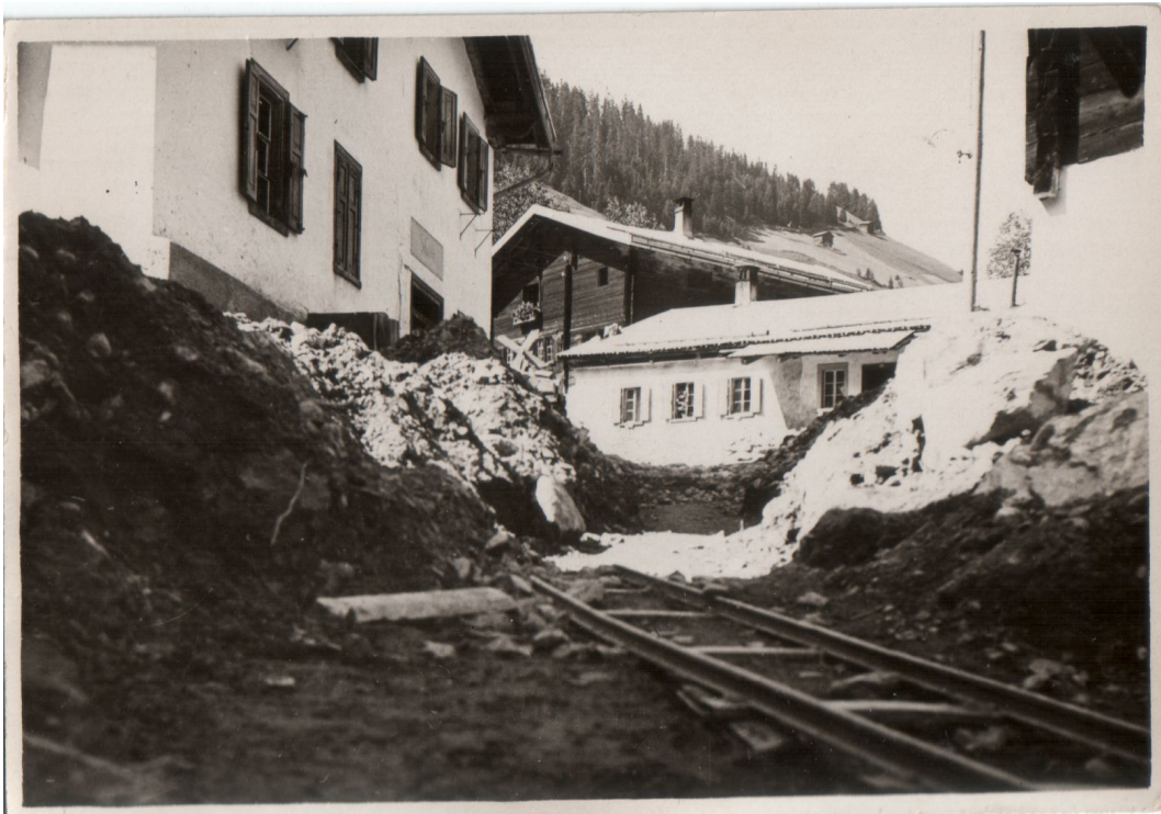
Illustration 1: Damage to property and the community after the flood.
