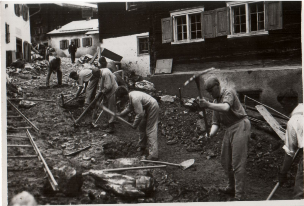
Illustration 3: Teamwork for rebuilding Safien.
