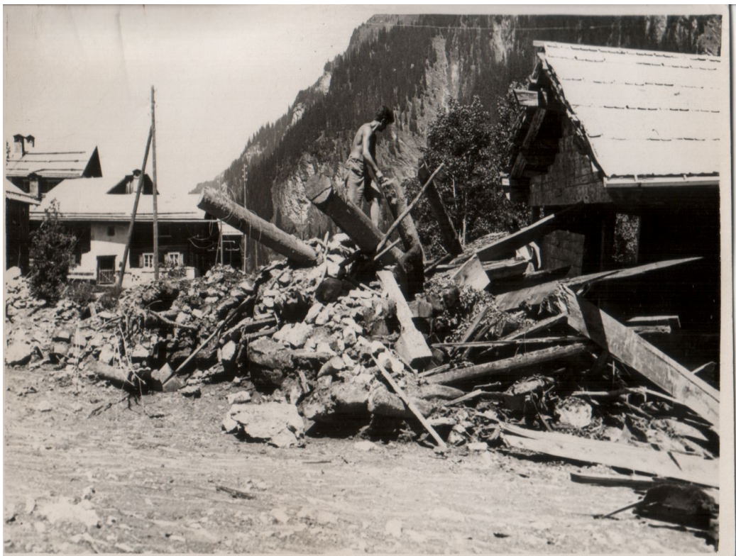
Illustration 4: Extent of flood damage to property.
