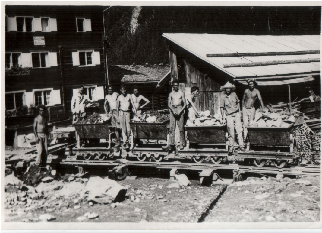
Illustration 2: Volunteers working to repair damage to property.
